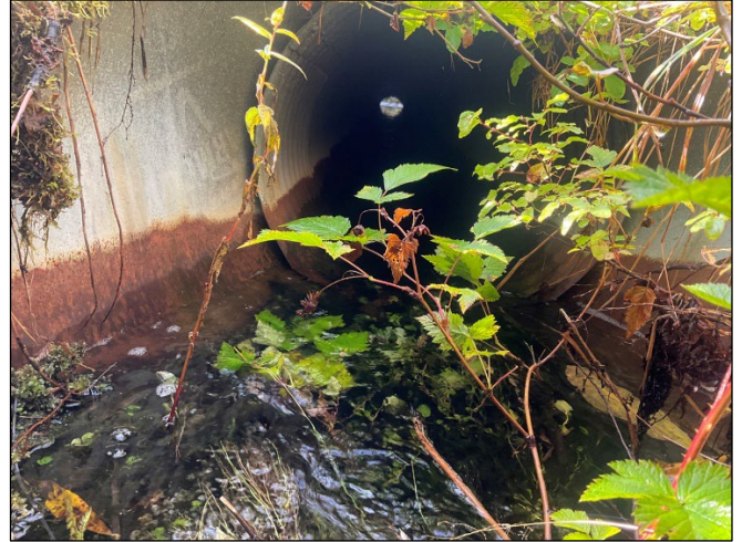
Figure 3.— Inside of culvert looking downstream.
